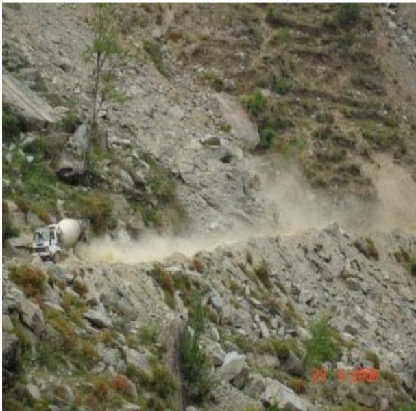
**Pic 7: Dust on the road to Raila, no water spraying**
