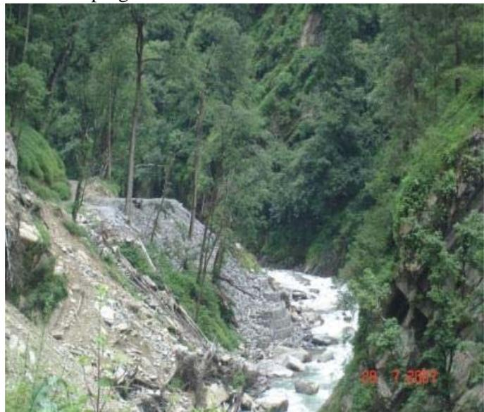
**Pic 4: Muck Spilling over broken retention wall near Majhan**
